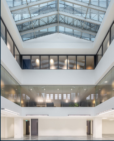
ABOVE: GROUND FLOOR UNIT RIGHT: INDICATIVE CGI OF TYPICAL UPPER OFFICE FLOOR
