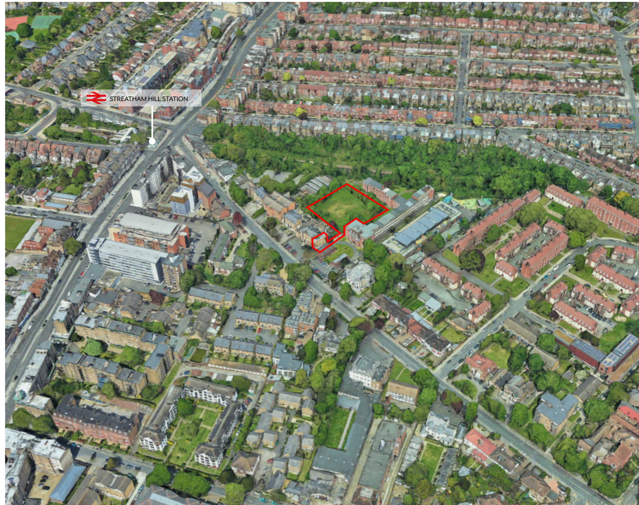
Aerial of site from South
